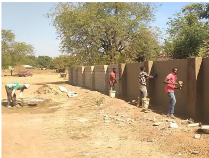
Beneficiaries of the Cash-for-work scheme rehabilitating the secondary school in Konduga
